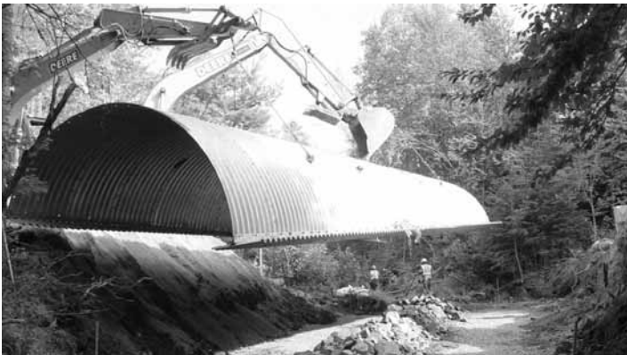
Installing the Rolfe Brook arch with stream diverted, 2008.
