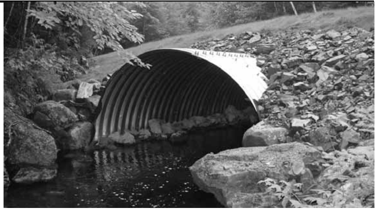
Scott Brook arch culvert, installed August 2008
