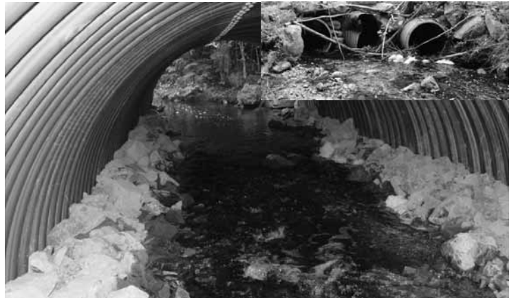
Scott Brook arch. Inset: culvert inlets before installation
